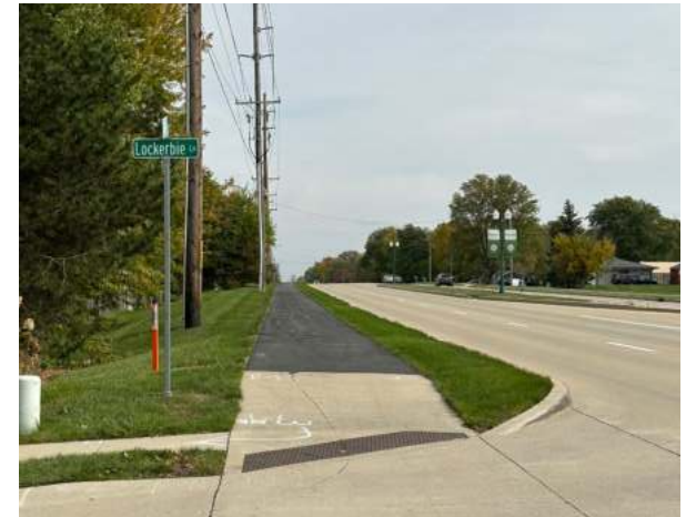
126th Street Existing Conditions
