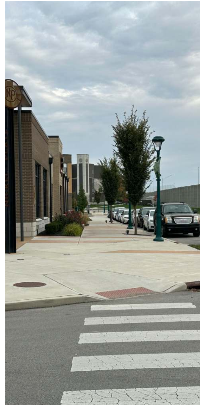
Existing Sidewalk on Lantern Road
