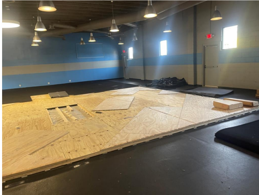
INTERIOR – FORMER FITNESS CLUB
