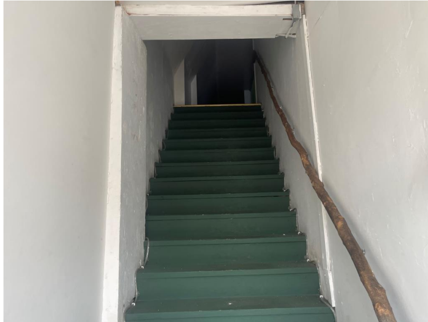
INTERIOR – STAIRWELL TO SECOND FLOOR
