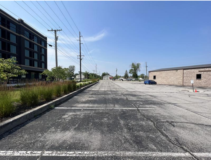
Facing south towards South Street from E. 116 th entrance
