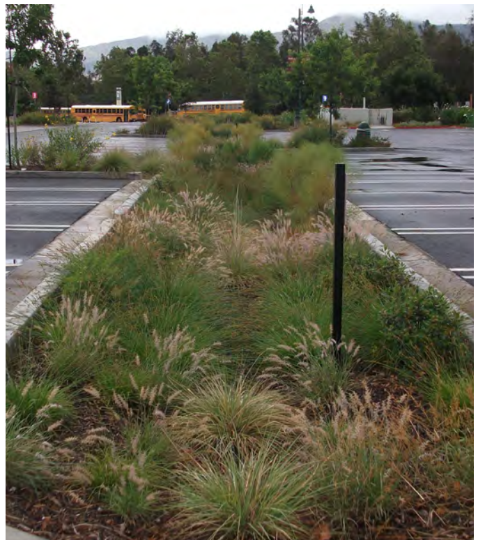
Stormwater planters, or bioretention swales, help to filter and reduce stormwater runoff.
