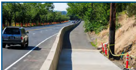
Multi-Use Trail with Physical Barrier
