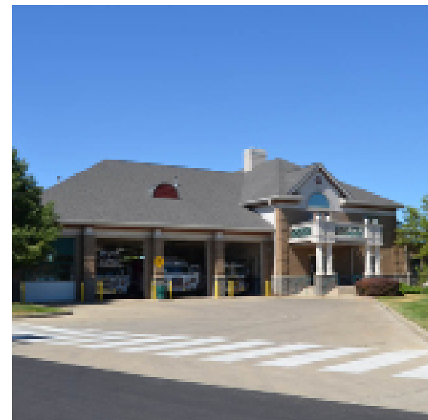
Municipal Center: Fire Station
