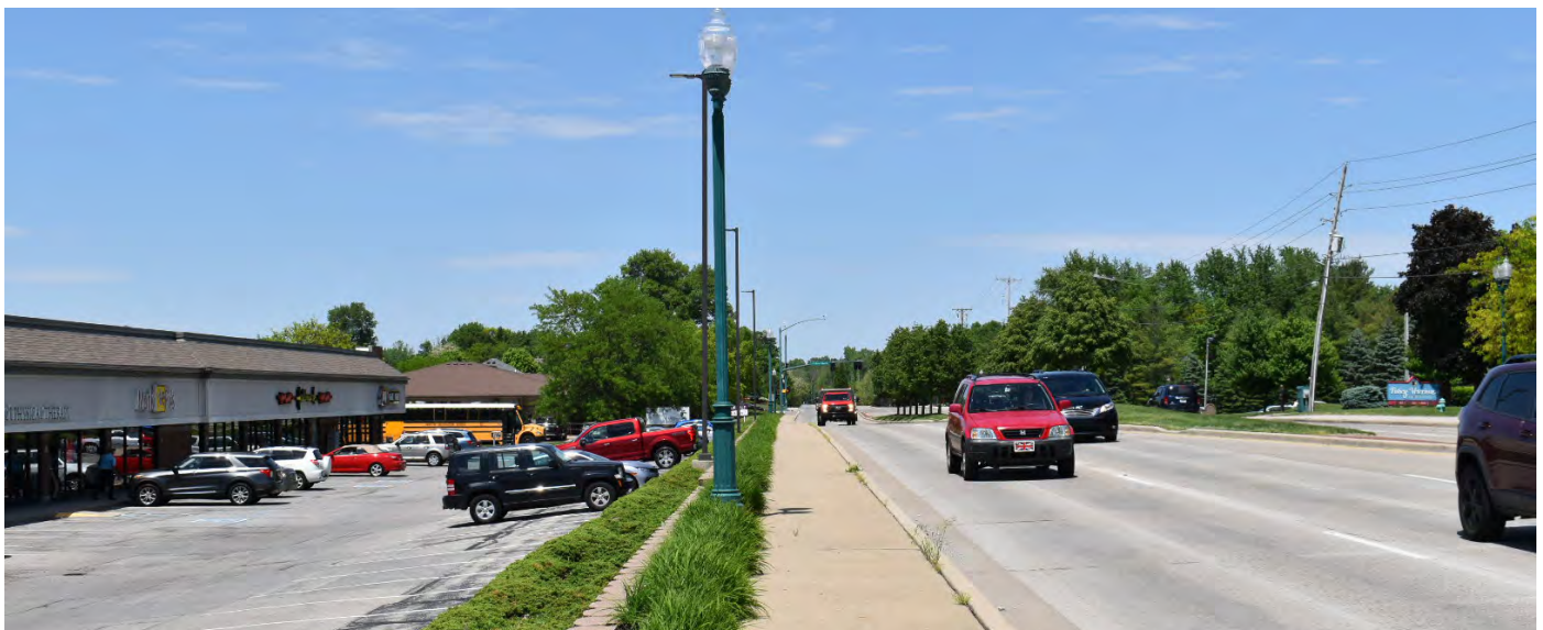
A typical sidewalk condition along the corridor.
