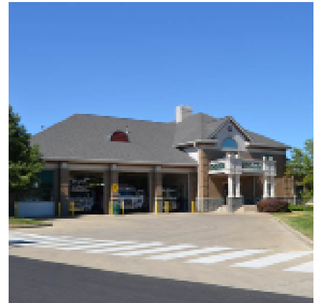
Municipal Center: Fire Station
