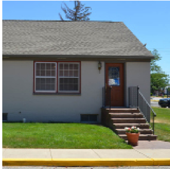
Existing single family home along Maple Street.
