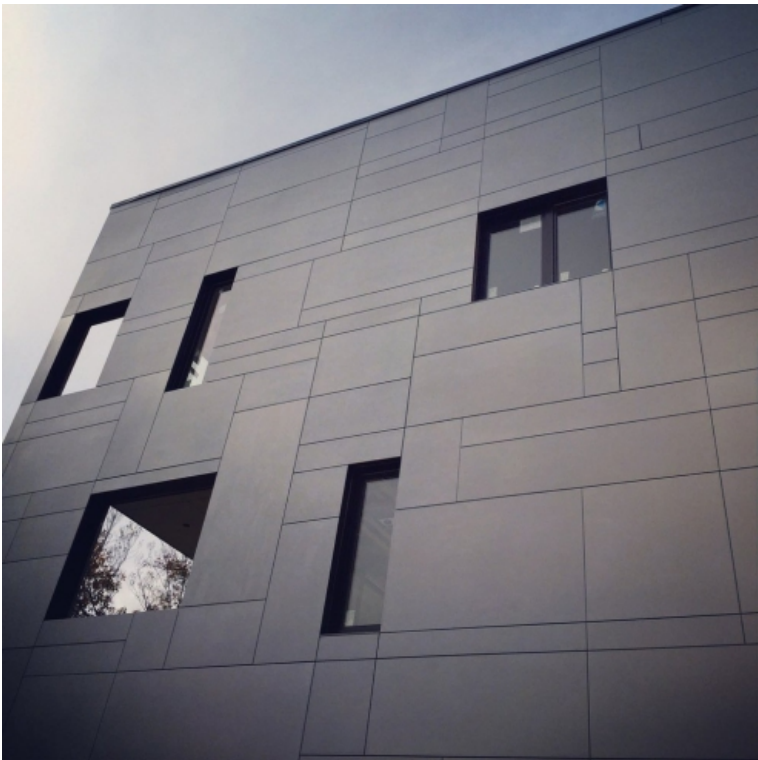
FIBER CEMENT PANELS HARDIE PANELS WITH METAL REVEALS
