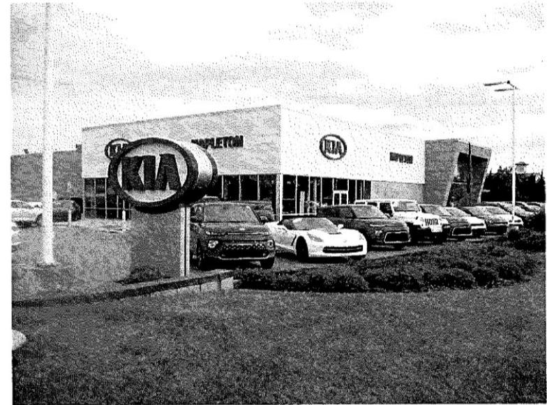
VIEW NORTHWEST OF AUTO DEALERSHIP – SIGN AND LIGHT IN TAKE
