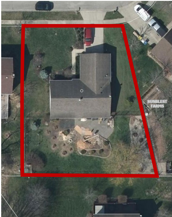
Aerial view of the property
