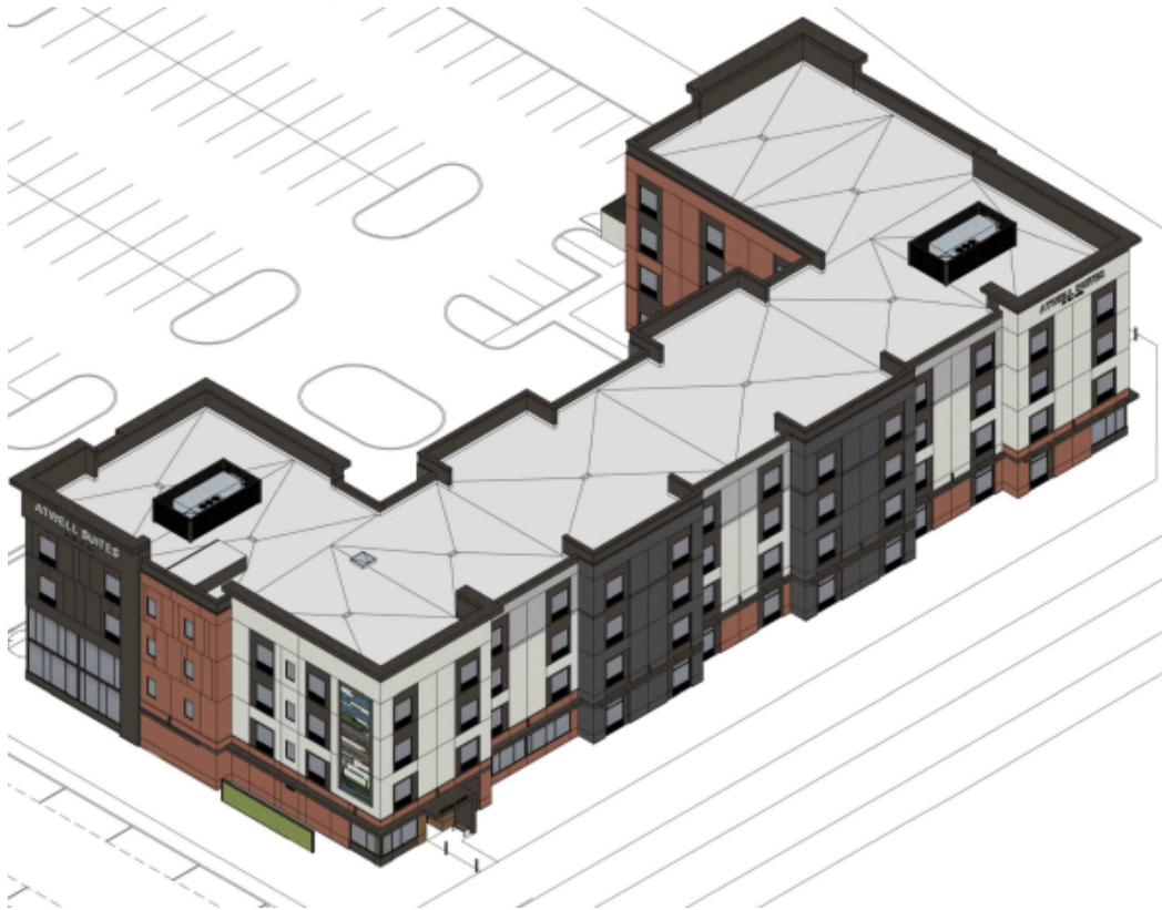
Southwest View, along E 134 th Street a new proposed public road
