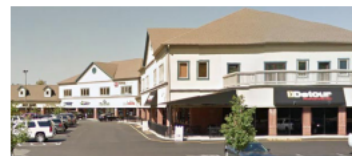
The restaurants and shops at the northwest corner of Fall Creek and Brooks School Road are an example of a neighborhood service center.
