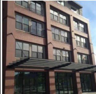
b. This building provides projections which articulate the building façade and provide temporary relief from inclement weather.
