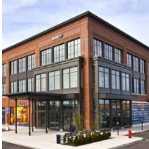
a. This building provides at least three (3) detailing elements that transition façade material changes and integrate pedestrian scale elements.
