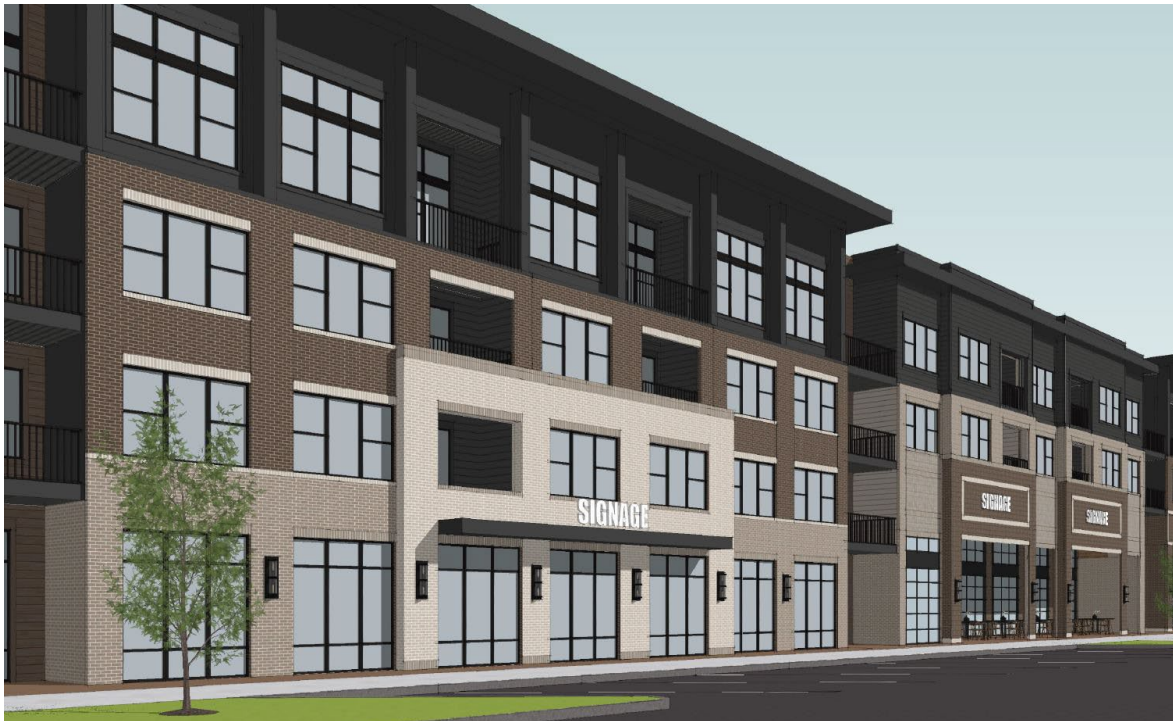
View from Stockdale Street of masonry details, light packs, and pedestrian scale.
