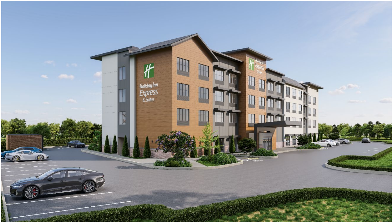
Southeast corner, looking northwest
