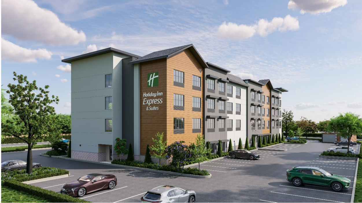
Northwest corner, looking southeast
