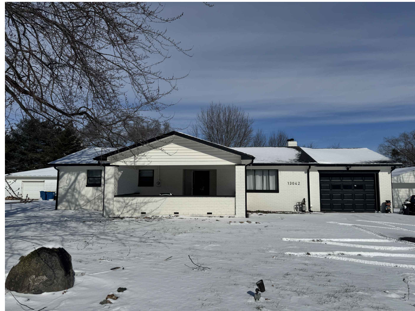
Front Elevation - South (Existing Conditions)
