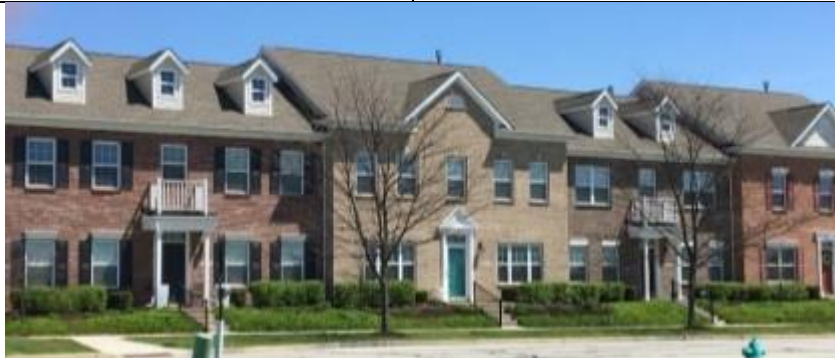
e. Attached residential developments shall provide a variation in roof heights to provide a unique identity to each unit.
