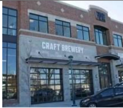
h. These roll-up doors are integrated into the building design.
