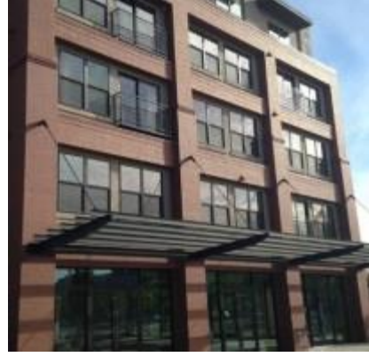
b. This building provides projections which articulate the building façade and provide temporary relief from inclement weather.
