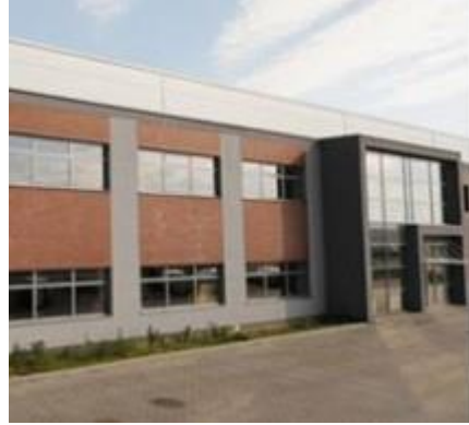
f. This industrial building uses concrete with qualifying materials.
