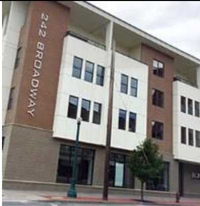
c. This building uses masonry as an accent material on the 1 st story or 1 st floor height.
