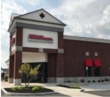
a. This roofline incorporates roofline and parapet variations.
