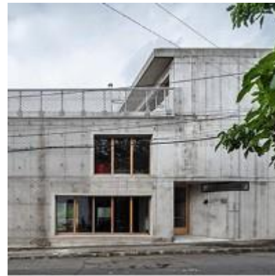
i. These untextured concrete panels are prohibited
