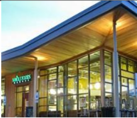
g. Reclaimed wood under the canopy is used here as an accent material.
