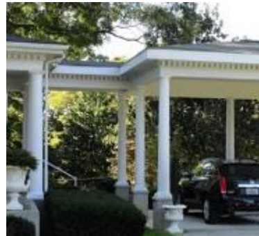
e. Carport is attached to the primary structure.
