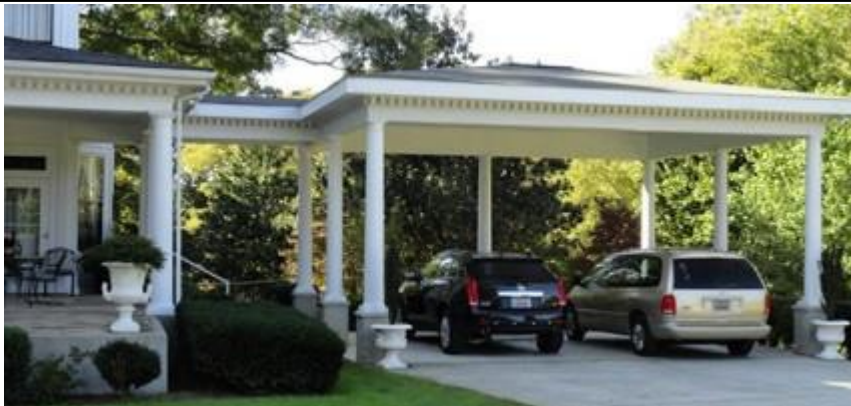
f. Carport is designed in keeping with the primary structure and utilizes the same materials and color.
