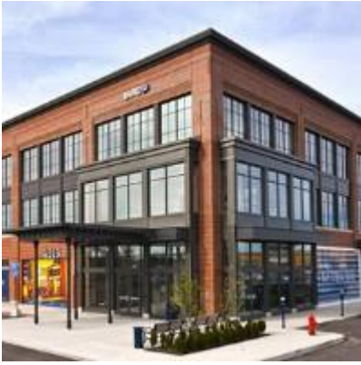
a. This building provides at least three (3) detailing elements that transition façade material changes and integrate pedestrian scale elements.
