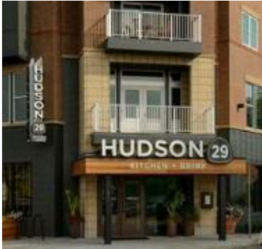
a. This building uses consistent material combinations, quality, and detailing.
