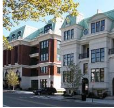
b. This building incorporates roofline and parapet variations.
