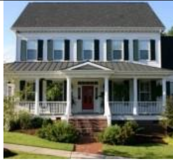
b. Roof massing is broken up into primary and secondary elements corresponding to architectural features.
