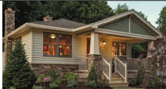
g. The use of .052 gauge vinyl siding may be allowed on single-family when it is combined with masonry at the water table line, two (2) architectural elements and a decorative entryway with a 12" min. door trim.
