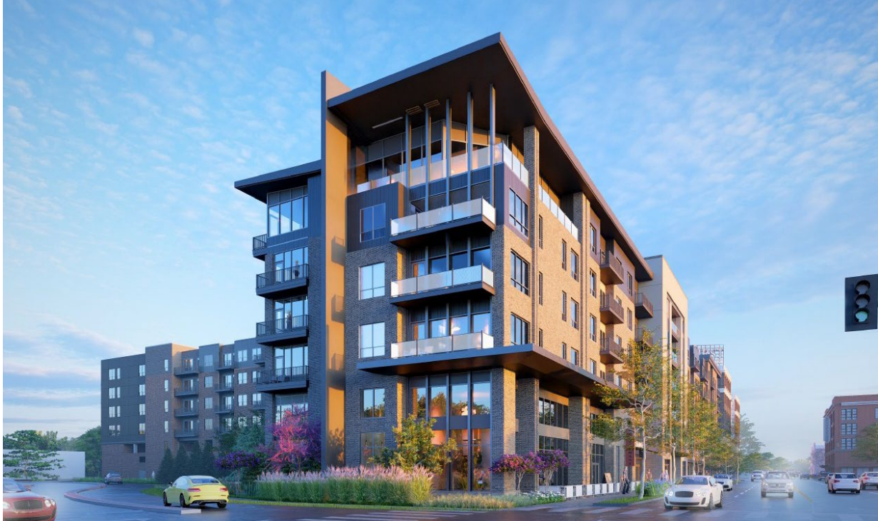
Northeast view along E 116th Street at Lantern Road
