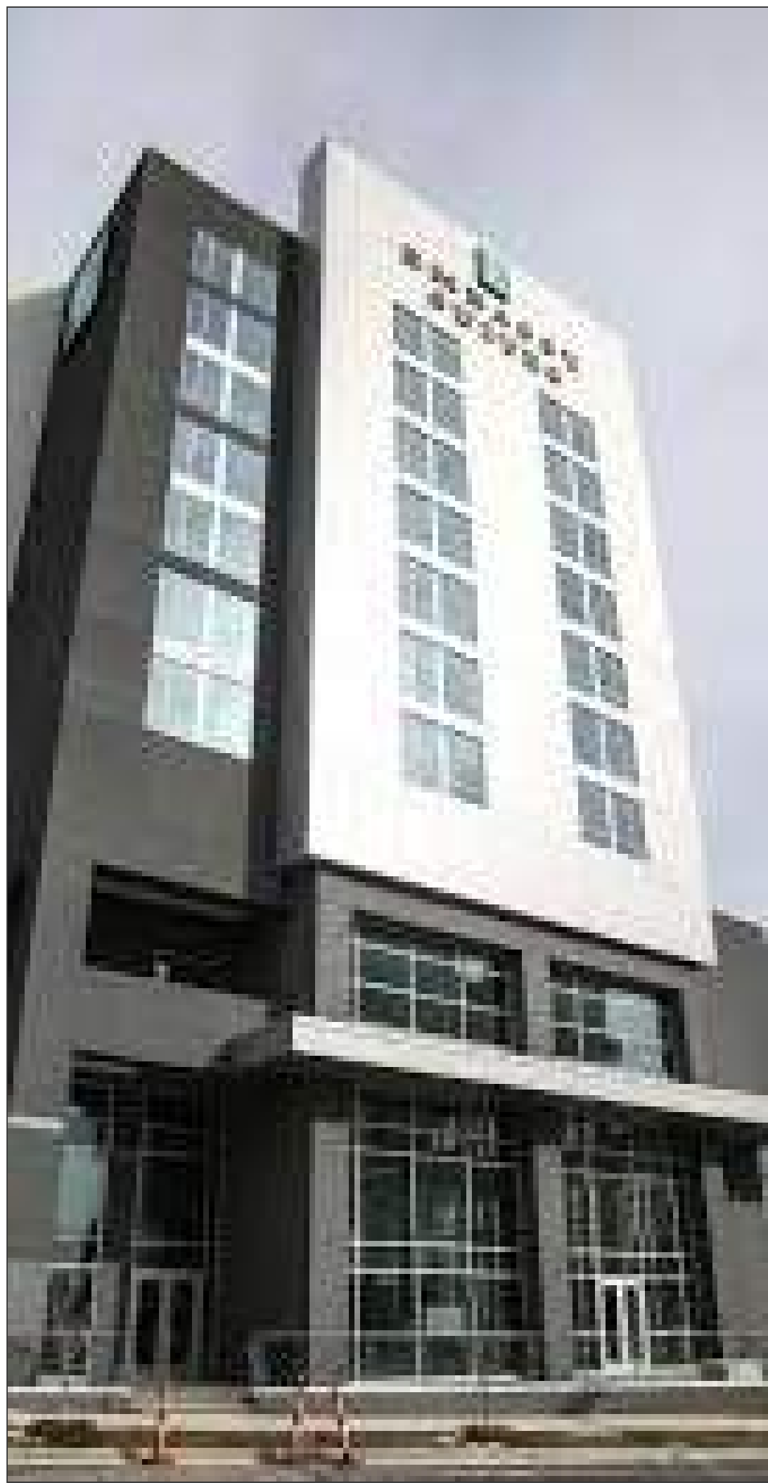
FACADE PLANES FLOATING ON MASONRY BASE
