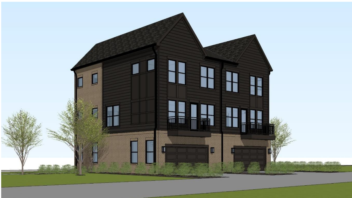
Rear Perspective of the Two-Unit Structure (Building 10)
