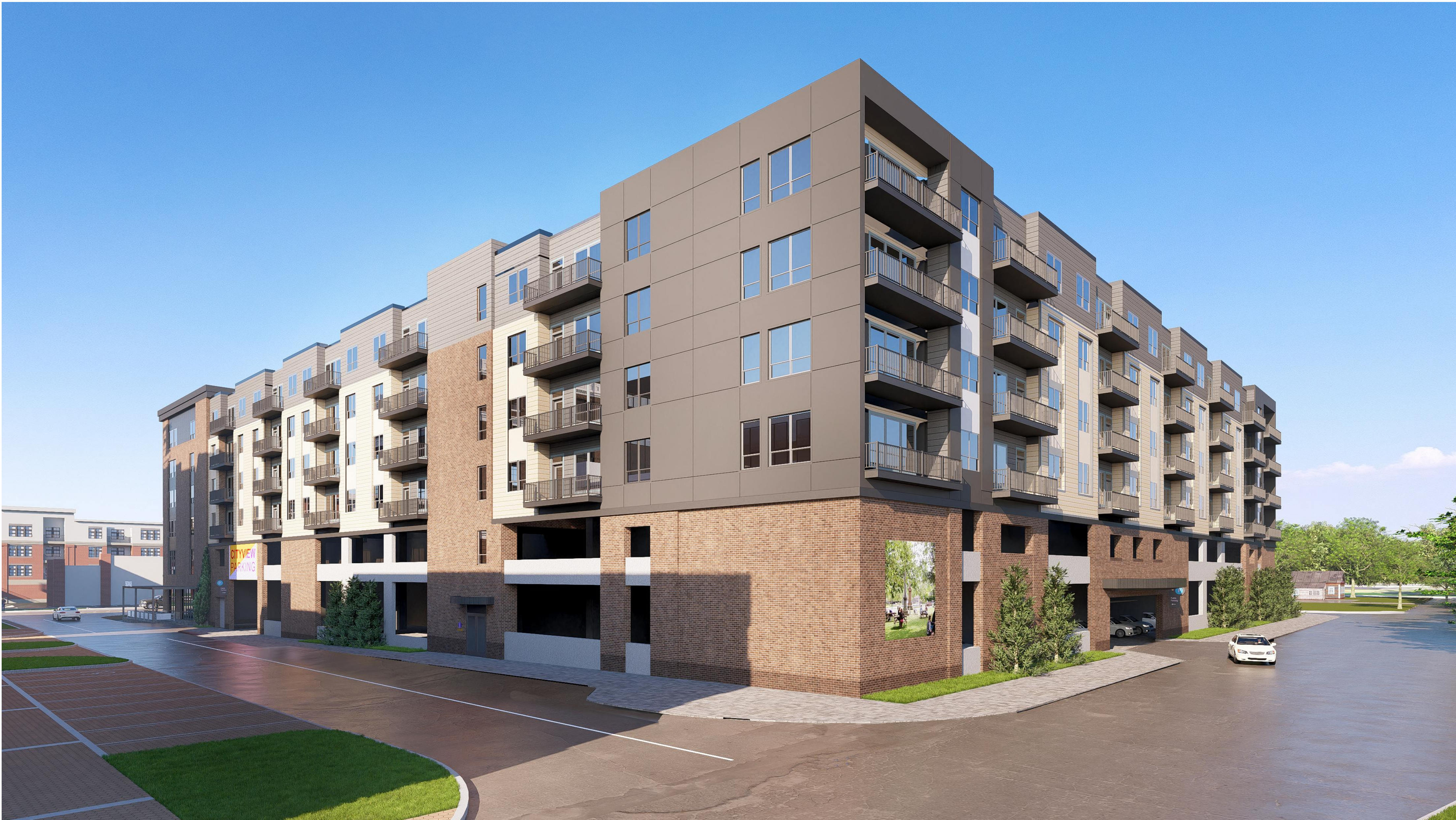
South West View from South St & Moore St
