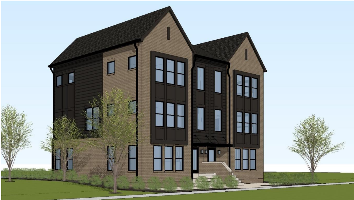
Front Perspective of the Two-Unit Structure (Building 10)
