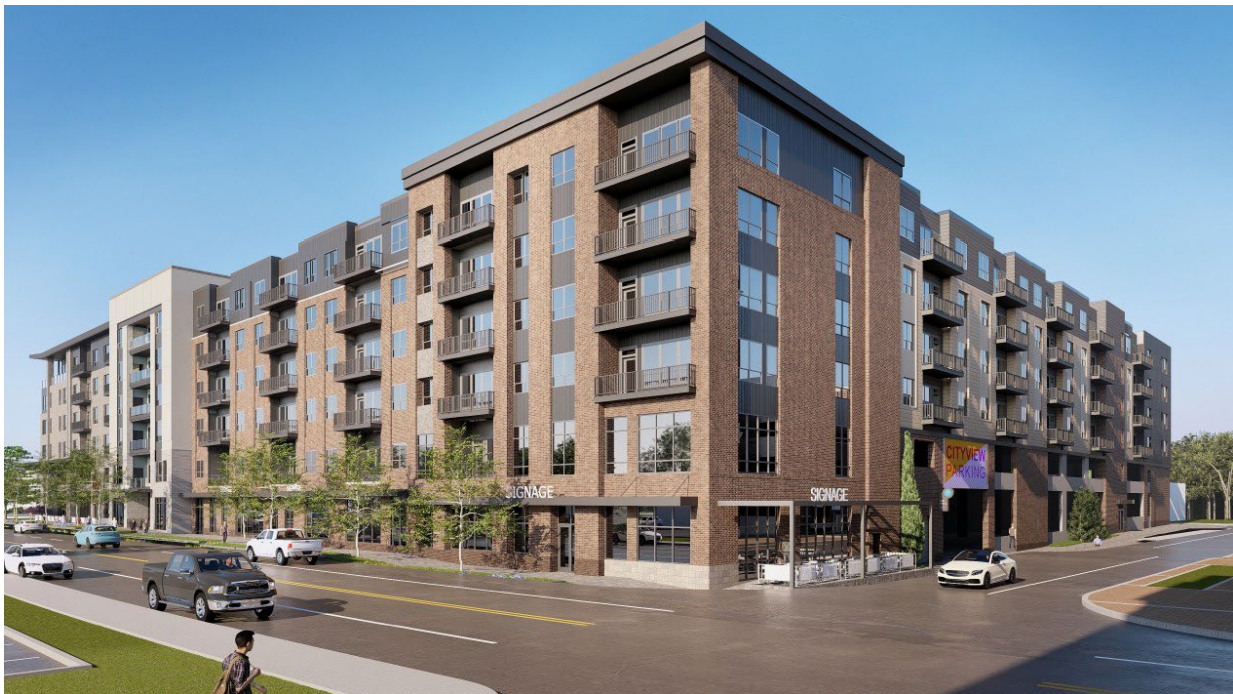
Northwest view along E 116th Street at Moore Street
