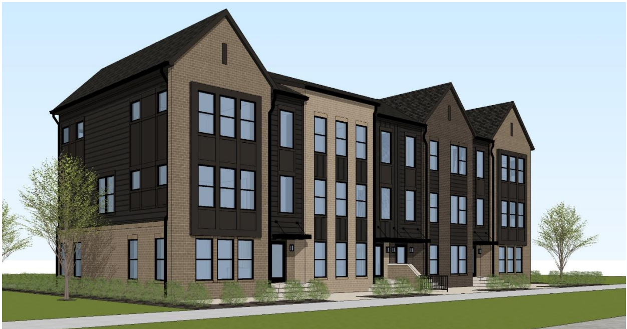
Front Perspective B of the Five-Unit Structures (Buildings 6 and 7)
