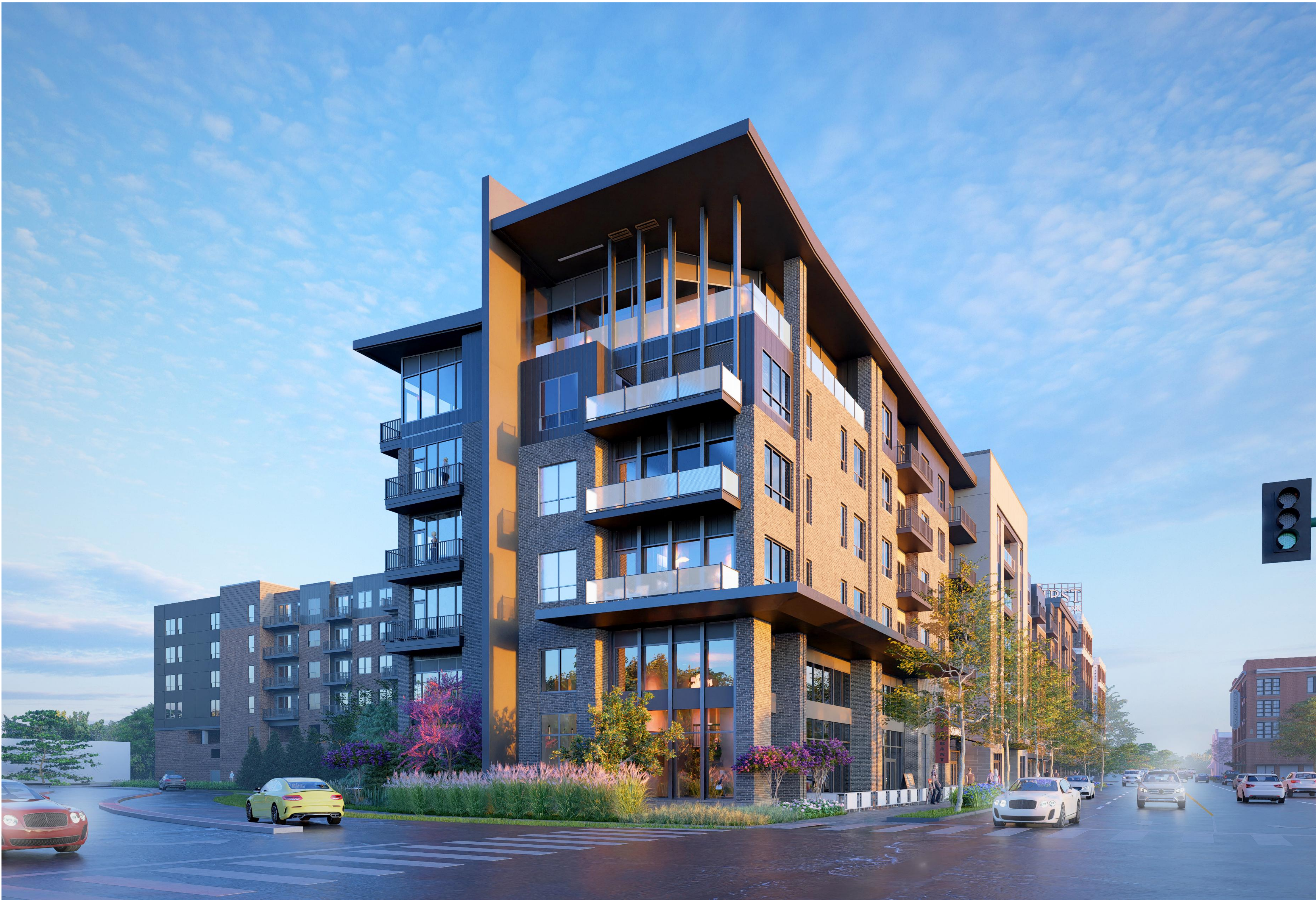
South East View from E 116th Street & Lantern Road
