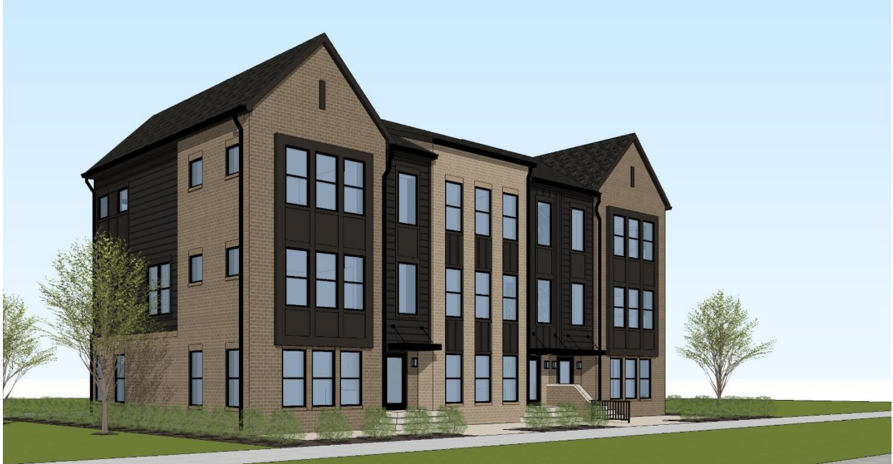
Front Perspective A of the Three-Unit Structures (Building 4)
