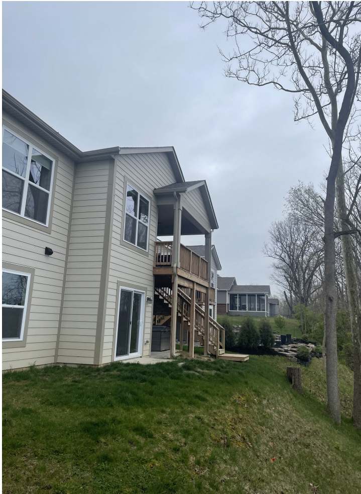
DEMO BOTTOM LANDING, HANDRAILS, AND PATIO DOOR STOOP
