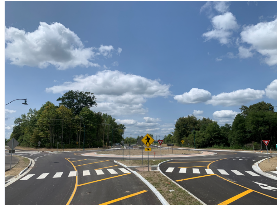
Newly constructed 126 th and Southeastern RAB
