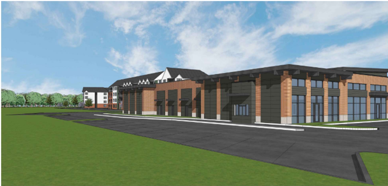
Building A from southwest
